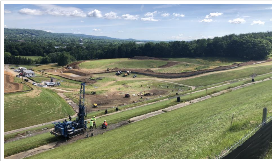
Installation of piezometers and abandoning existing instruments at the North Dam
