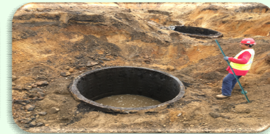
Removal of contaminated leaching pool/drywell
