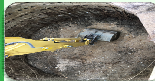
Removal of contaminated from drywell
