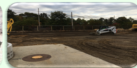
Backfilling and grading
