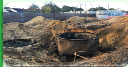
Removal of contaminated leaching pool/drywell
