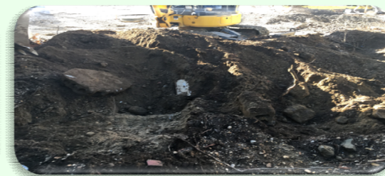
Excavation of contaminated soil to the extent feasible
