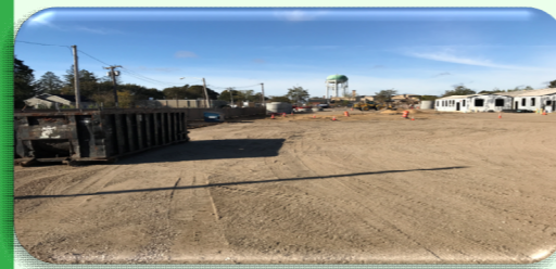
Pre-remediation demolition of structures
