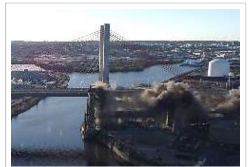
Blast demolition of a bridge near monitored LNG tank
