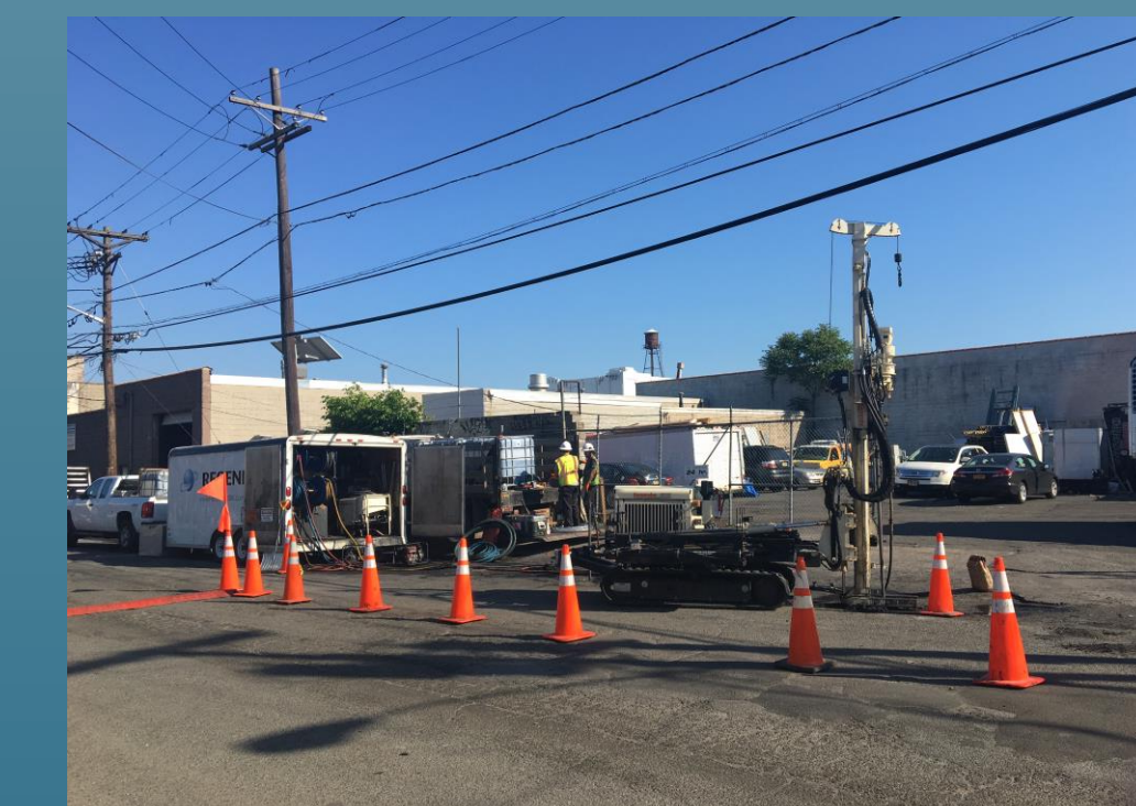
Bio-barrier injection between Area 2 and 3
