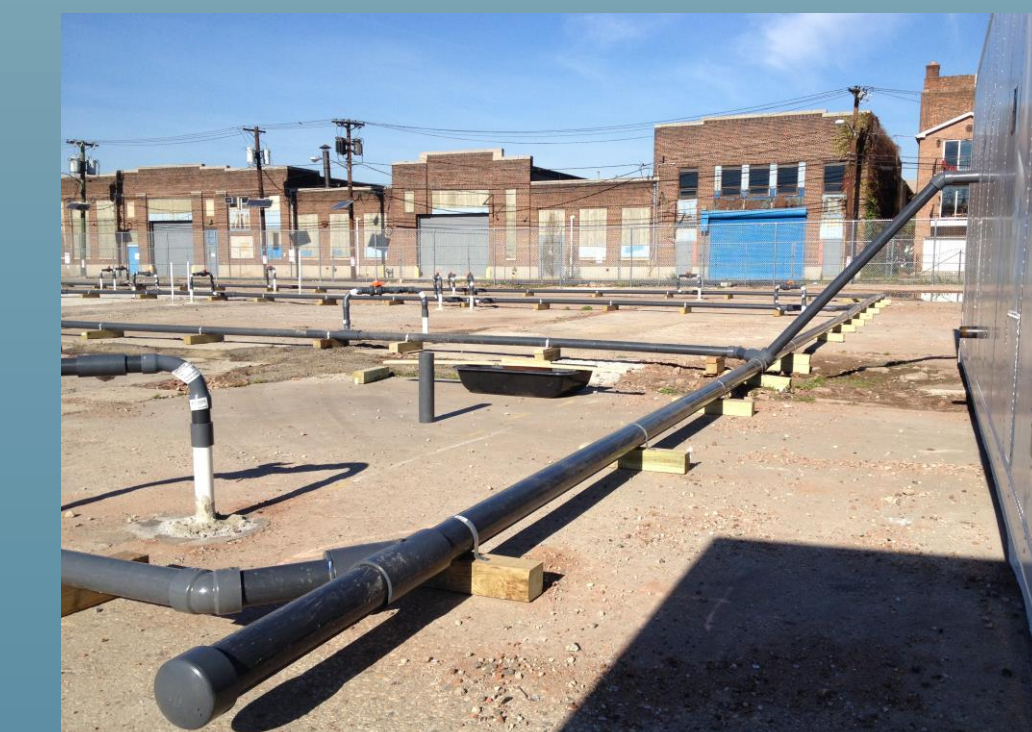
SVE system operated in Area 1
