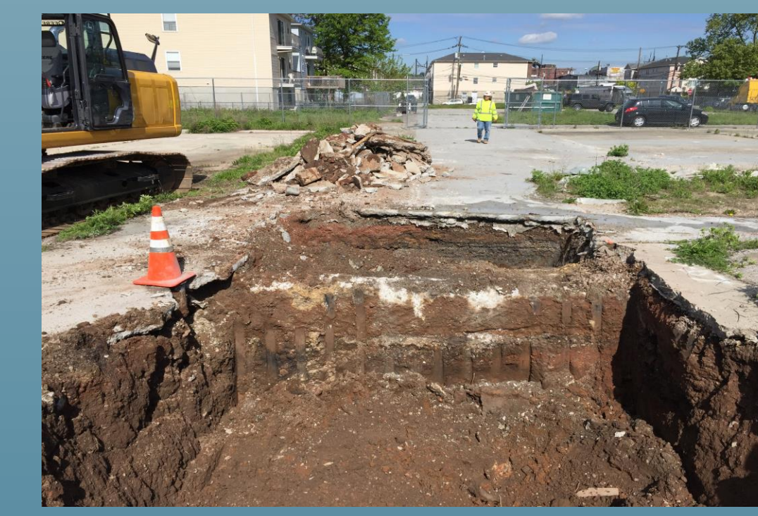
Soil Excavation in Area 1
